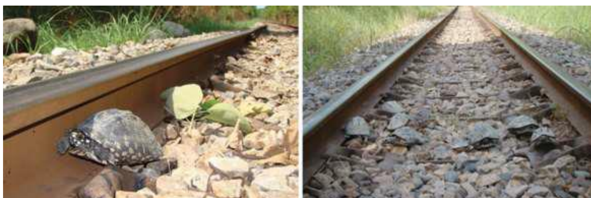
Figure 7.2 Barrier effect of the railway track for turtles (Source: Dorsey et al., 2015)
